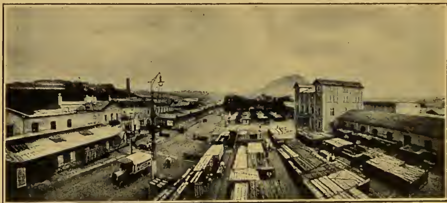
FIG. 4.—General View of the Works at the Apollinaris Spring.
